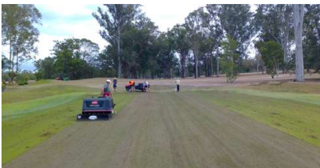
GREEN RENOVATIONS UNDER WAY
